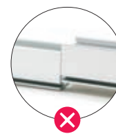
parallel vertical misalignment
